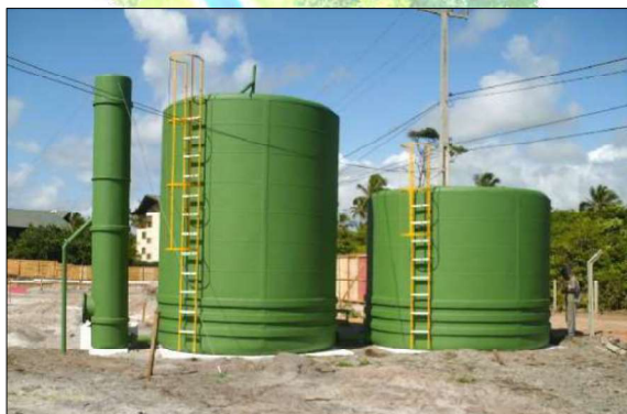
Figura 70 – Reator UASB
